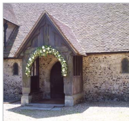
North door and timber porch
