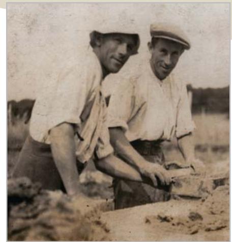
Bill (left) and Harold Pycroft making bricks
